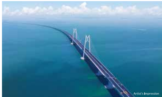
Hong Kong - Zhuhai - Macau Bridge
